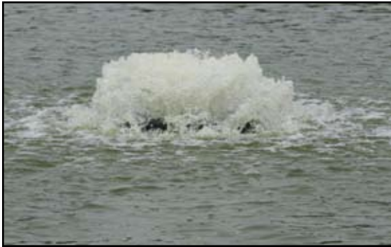
A surface spray aerator at work
